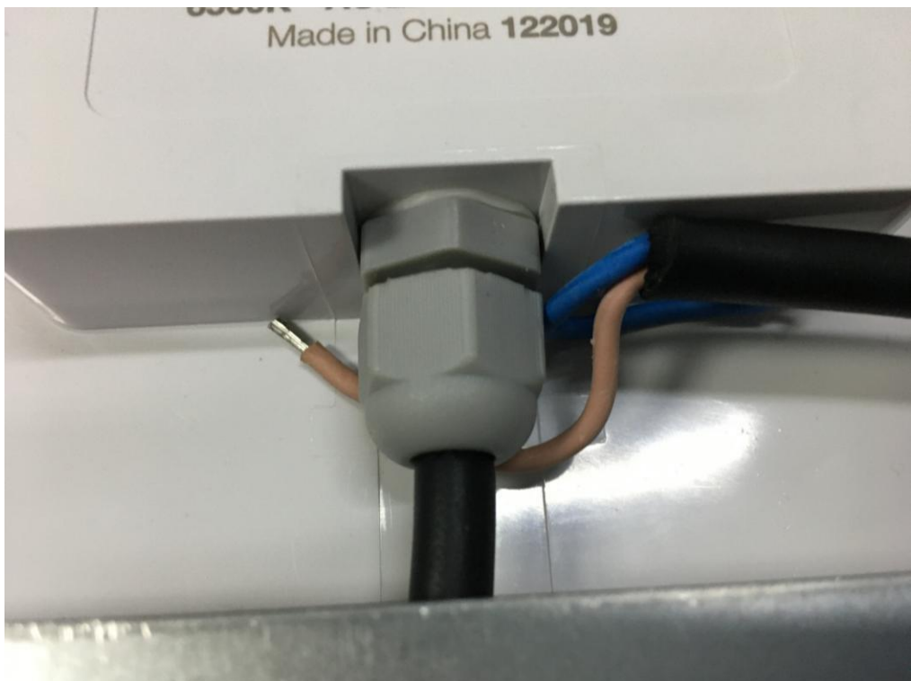
Figure 4. General view of MT60179
